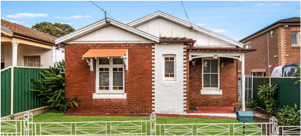
Figure 2: View of Subject Site from Taylor Street
